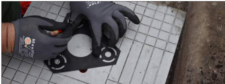
Use the charger's template to determine drill hole pattern. The ChargePoint CT4000 template is shown in the image above.
