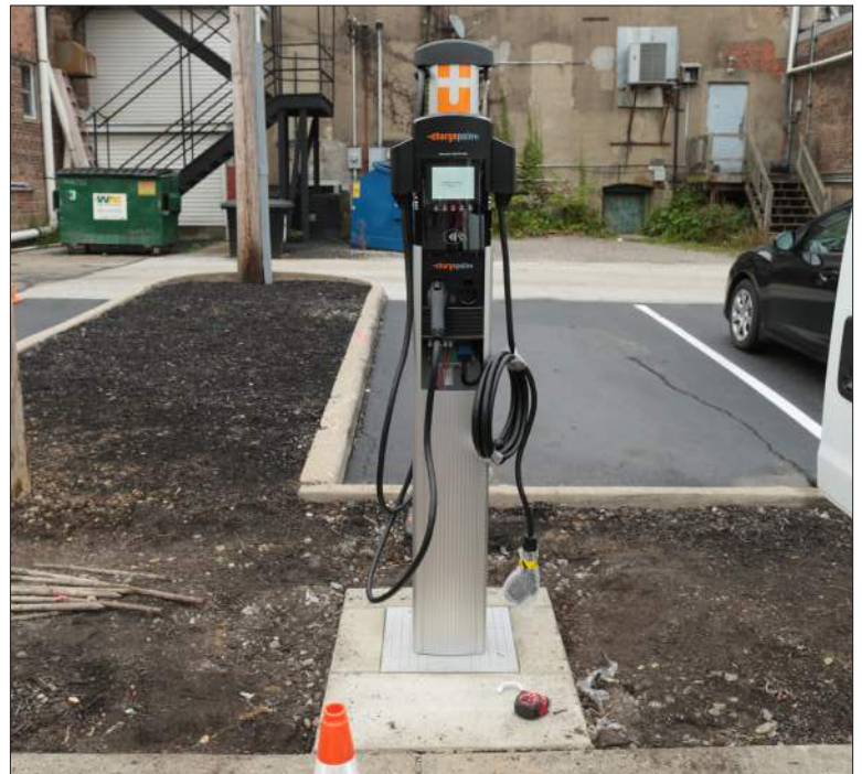
Completed foundation installation, with an attached charger.
