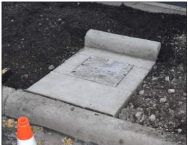
Completed foundation installation.
